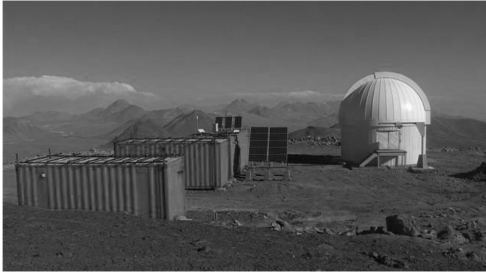
Figure 3. A full view of the summit facilities. From right to left, the telescope dome, the operation container, the storage container, and the generator container are seen.
