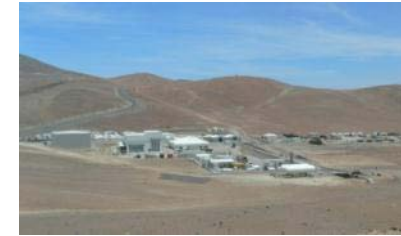
The Paranal observatory (Chile) - 8-m telescope x 4 units - One of the largest observatory - Power consumption is 2MW.
